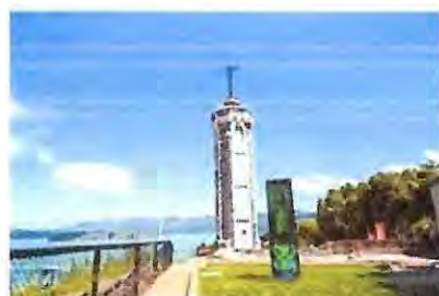
The rebuilt Lyttelton Timeball Station in November 2018
