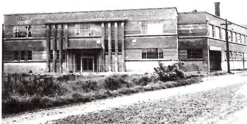
The building as it appeared when new in 1954. Image courtesy of Naylor Love.
